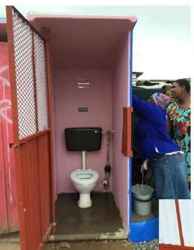
**Drainage improvement**A variety of wastewater drainage ideas were put in place to be trialed. Top and right pictures show the ground drain has been capped and filled with the new tub drain installed. Bottom left picture shows the new tub drainage working and the newly improved ground drain blocked. These alternatives will be assessed and reviewed in mid 2014 using thel data collected on the volumes of water being drained.
