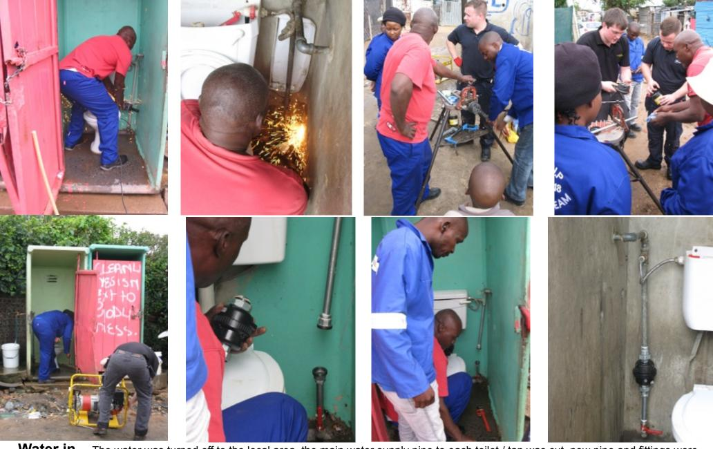
**Water in** — The water was turned off to the local area, the main water supply pipe to each toilet / tap was cut, new pipe and fittings were made to install an isolation valve for water control and a water meter to record use. Because of the high demand on each toilet, the existing toilet cistern was reconnected in the short term, and the mains water turned on to allow use.
