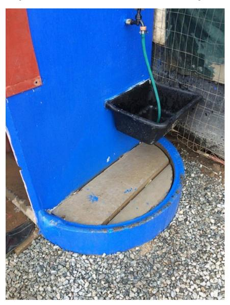
**General improvement**Gravel was used to infill erosion and improve ease of access to the toilets and tap points. The gravel also helps maintain drainage and water flow around the toilet units. WASSUP began placing their brand on the improved toilets - linking their work to improved function.
