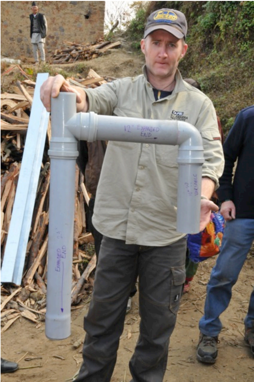
Detail of the fabrication and fitting: the completed pipework for Types A (shown) and B
