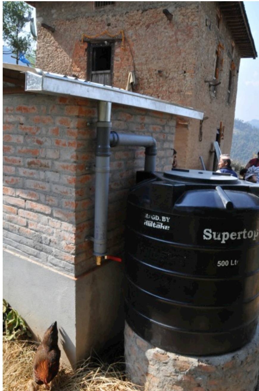
Type B diverter, with valve, completed
