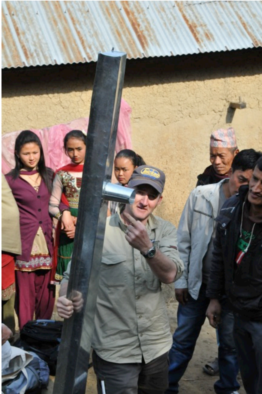
Detail of the fabrication and fitting: the completed gutter and spout
